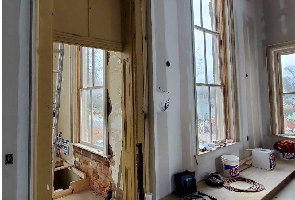
Finishing paint touches/finished carpentry wrapped around door casing to match existing.
